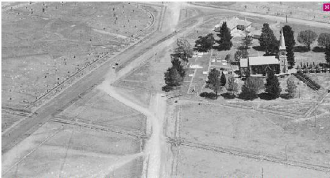
When the Scott's Crossing bridge was completed in January 1929, a major road improvement program was underway. That may explain the two machines on the road opposite what is now the Anzac Parade entrance to St John's graveyard. For Mark, this is another of the 'little-known images' of the railway (foreground) discovered recently. It was catalogued as, 'Aerial view of a cathedral, Canberra, ca. 1920s'.
