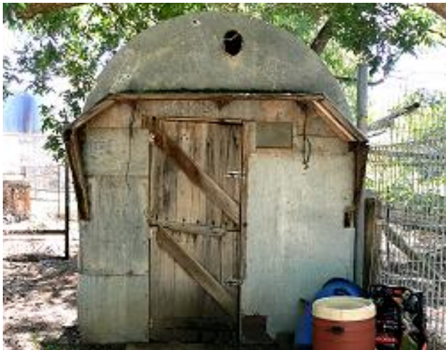
Sheds attached to or associated with the "Majura House" woolshed, some making good use of half-tanks as roofs c.1950s; turkey pens at upper right (Mark Butz March 2023)
