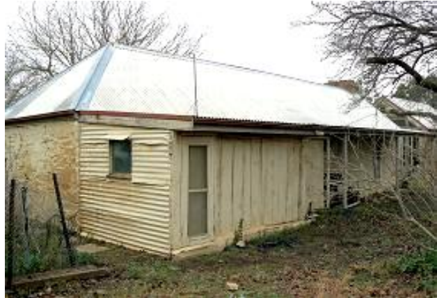
Skillion roofed vertical slab extension (Mark Butz June 2021)
