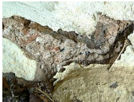
'Majura House' stone cottage (western side); wall details visible through flaking paint, showing stonework and mortar (Mark Butz March 2023)
