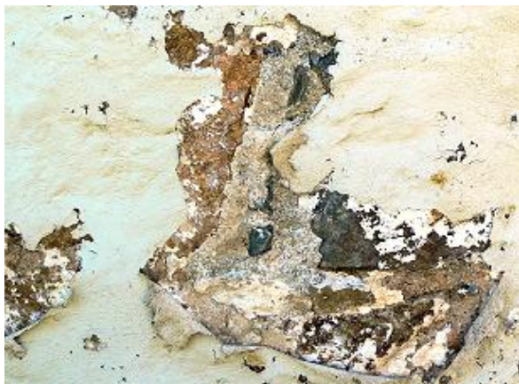
'Majura House' stone cottage (western side); wall details visible through flaking paint, showing stonework and mortar (Mark Butz March 2023)
