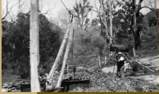
Using a bush gantry to load leaves into the still.
