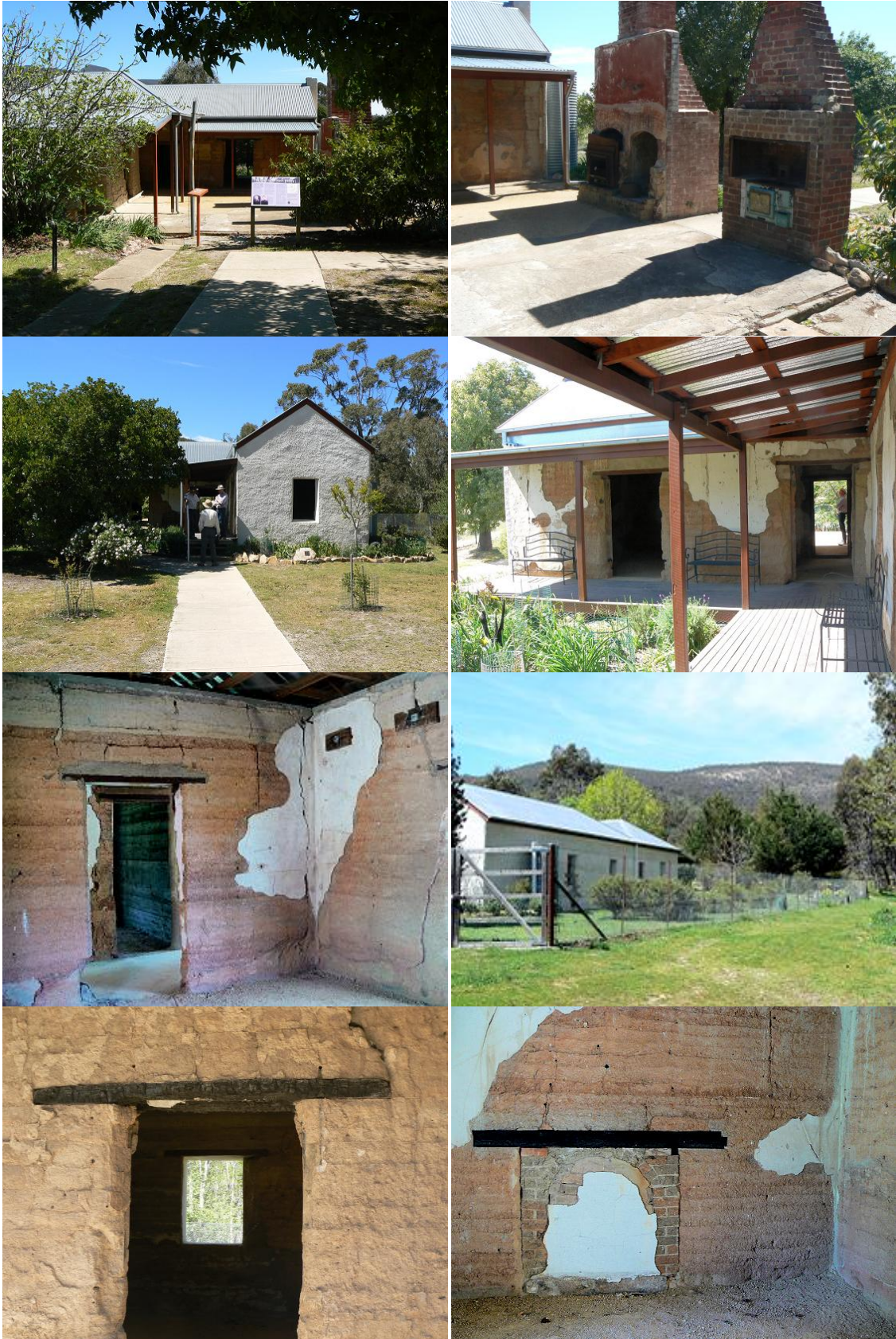
Collage of views, showing stabilisation measures, extant chimneys, internal exposure of pisé and plaster construction, and charred lintels, jambs and mantels (Mark Butz - Nov 2019 & Sep-Oct 2020)
