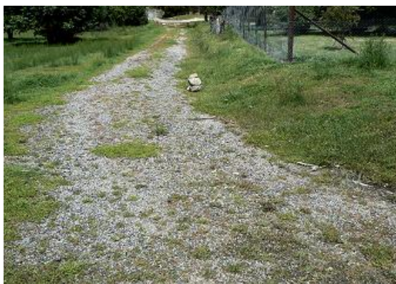
Intrusive and inappropriate ‘metal’ surfacing on the side access (left) and northern part of the car park - remediation with decomposed granite would approximate better the look of the pastoral era (Mark Butz – Nov 2020)
