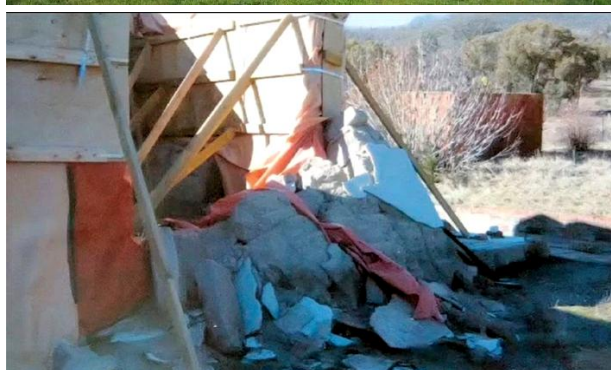
Right: Part of a wall collapse (1895 section) while awaiting decisions on the building's future (capture from TAMS video)
